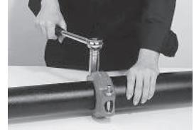
Check the pipes ends. The groove must be of uniform depth and its dimensions conform to QUIKCOUP® specifications. Both pipes end should be free of indentations, rust or roll marks from the end of pipe to the groove.
