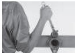
■ Check the pipe surface. The hole must be cut or drilled on centerline of pipe and in dimensions conform QUIKCOUP® specifications.
