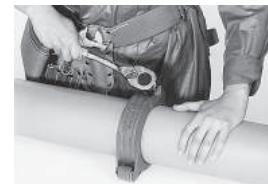
Check the pipes ends. The groove must be of uniform depth and its dimensions conform to QUIKOUP® specifications. Both pipes end should be free of indentations, rust or roll marks from the end of pipe to the groove.
